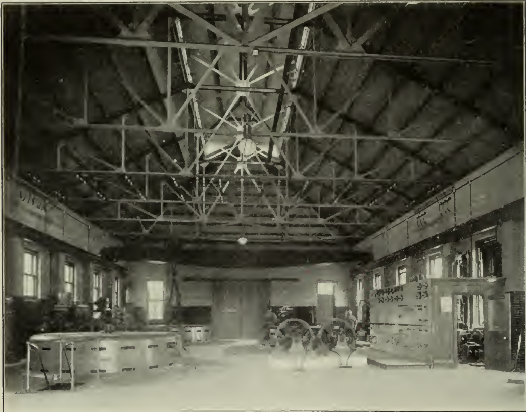
INTERIOR OF PUMPING STATION NO. 6.
